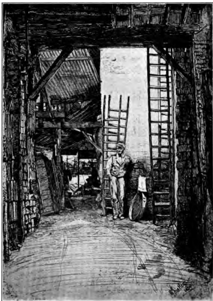
THE LIME BURNER (ETCHING).
